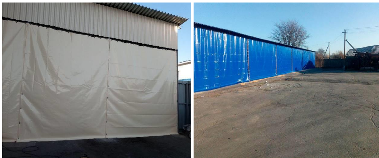
Fig. 1. Equipped storage shed for harvesters.
