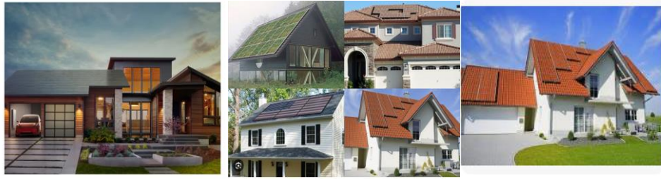
Figure 1. Tesla Solar Roofing
