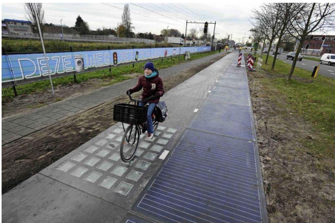
However, after 6 months of tests, SolaRoad was still recognized as an effective technology for was able to give a little more than expected 70kW of electricity per square meter. A year later the results (9800 kWh) compared with the results of solar panels of the same size, but mounted on the roof, and yet acknowledged that "high-
