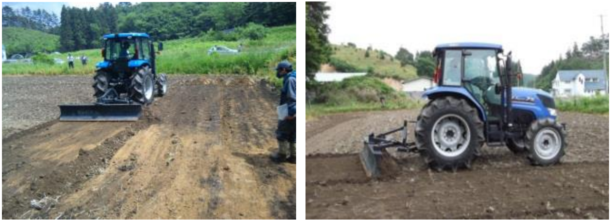
Fig. 79. Removing of topsoil in area contaminated by radionuclides (Japan, 2011).
