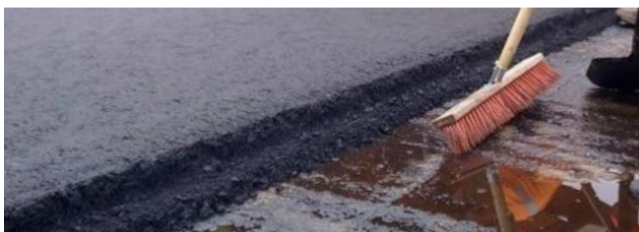
Fig. 2. Asphalt concrete floors
