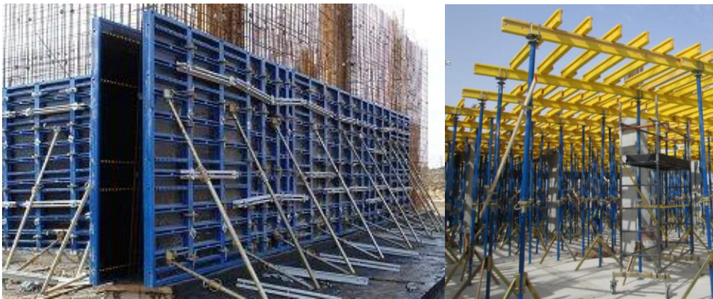
Figure 4 – Example of the VARIANT formwork system
