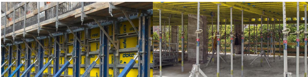
Figure 2 – Example of the DOKA formwork system
