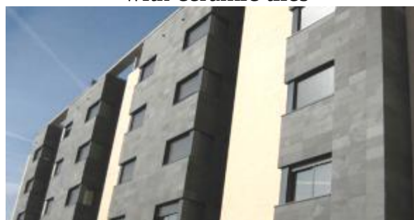
Fig. 7. Facing with facade porcelain stoneware
