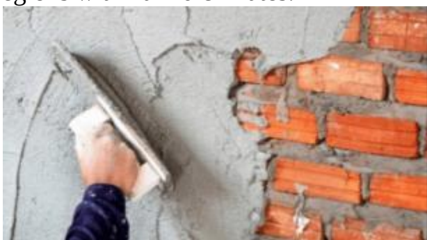
Fig. 2. Plastering the facade
