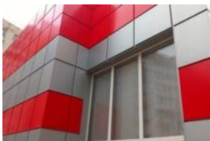
Fig. 6. Facing the building with facade cassettes
