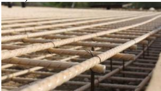
Fig. 3. Example of composite reinforcement application
