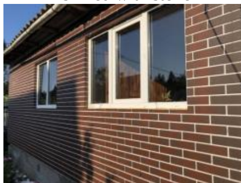
Fig. 5. Facing the facade with ceramic tiles
