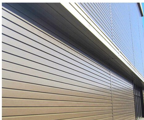
Fig. 4. Facade decoration with siding
