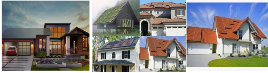
Figure 1. Tesla Solar Roofing
