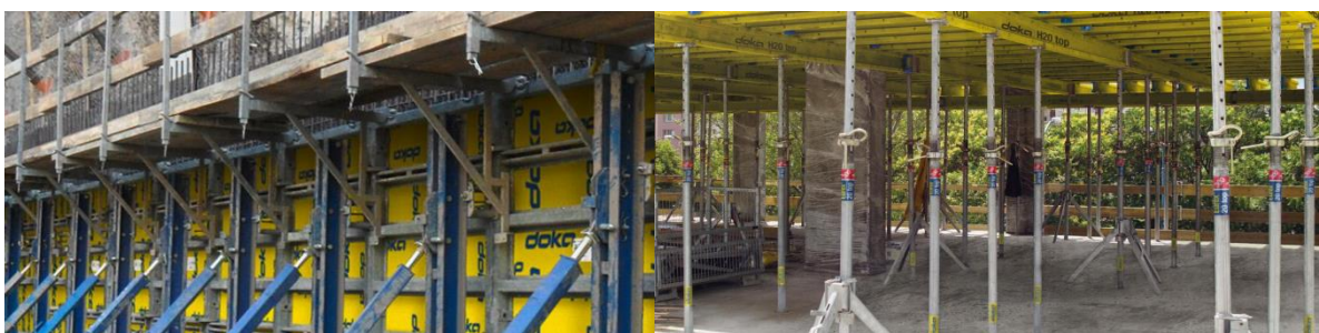
Figure 2 – Example of the DOKA formwork system
