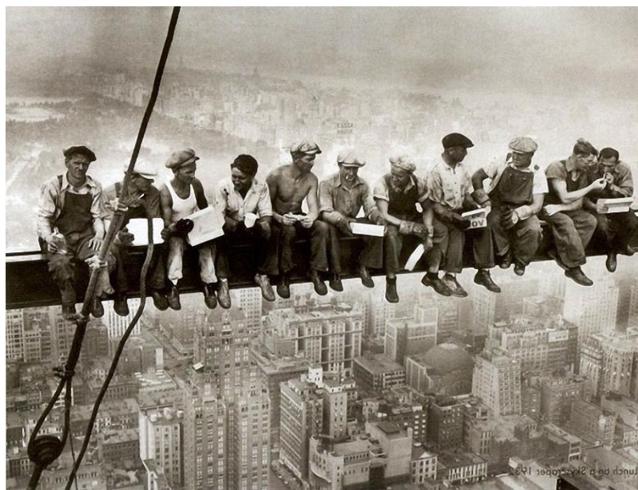
Figure 1 – Riveter on a steel beam of a steel frame September 29, 1932
