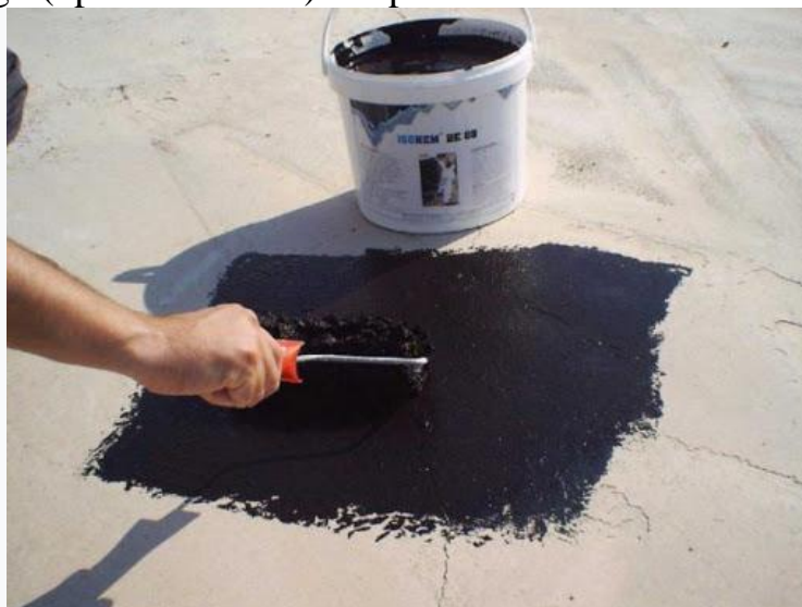
Fig. 1. Manual application of bituminous mastic
