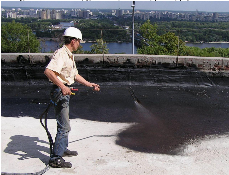
Fig. 2. Mechanical application of bitumen mastic
