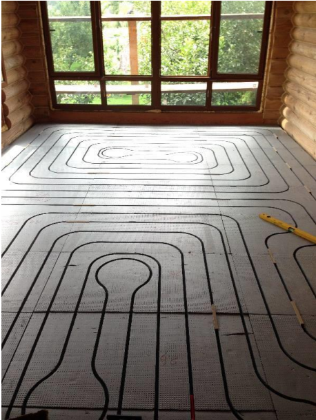
Figure 2 – Example of an electric system
