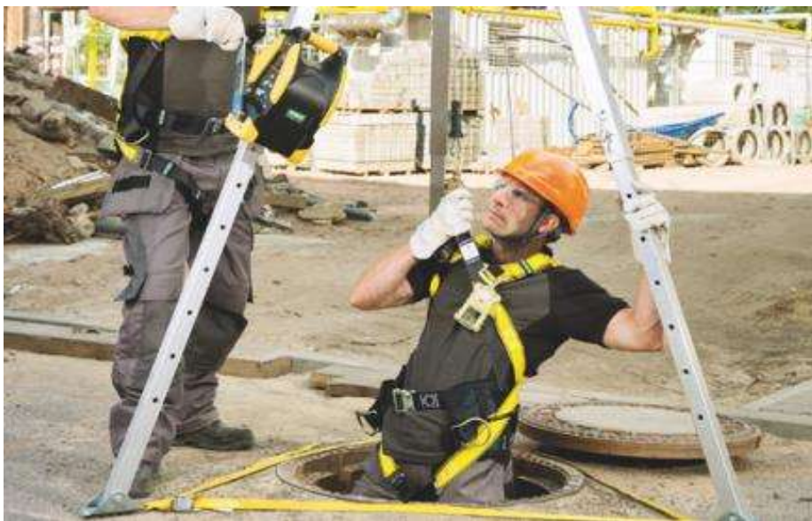
Fig.1. The work in closed containers and spaces
