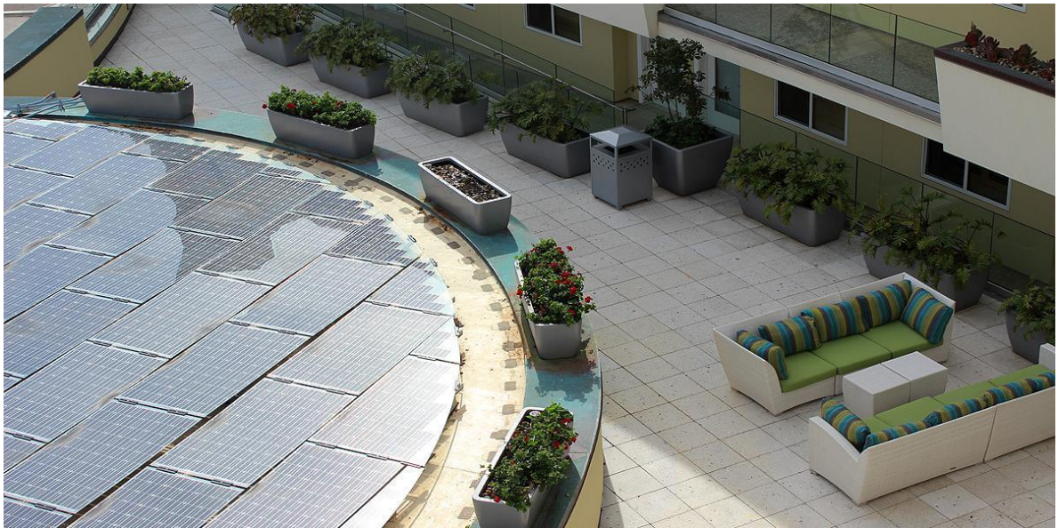
Fig. 3 Boutique hotel with photovoltaic roof
